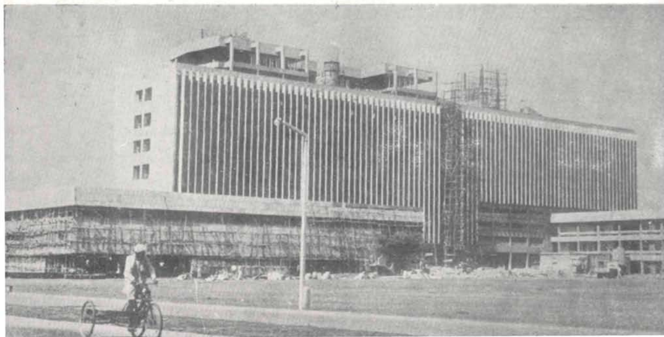
Multistorey block, a'most ready, partly occupied
