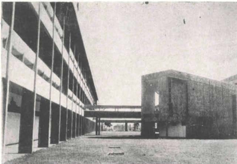
An engineering block
